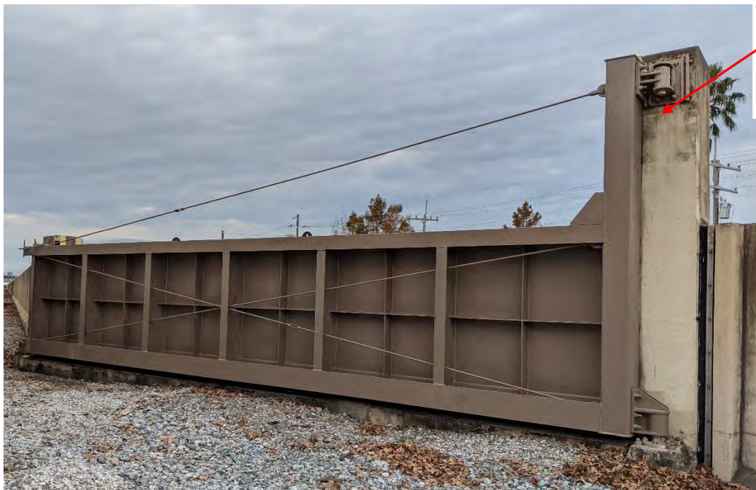
Figure 7.3 – Swing Gate with Large Length-to-Height Ratio
