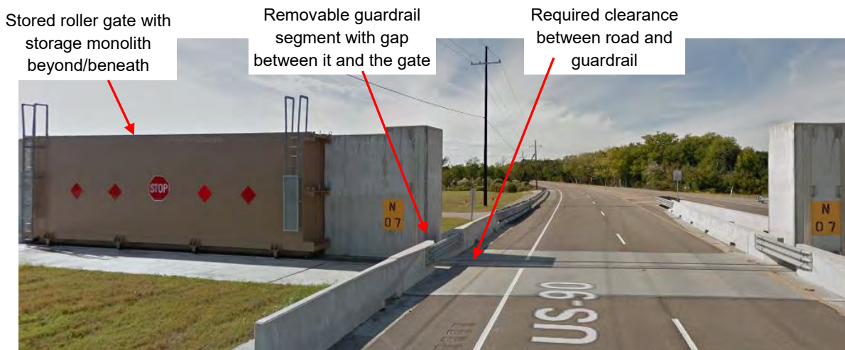
Figure 7.2 – Roller Gate with Removable Guardrail Arrangement
